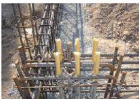
Setting up anchor bolt
