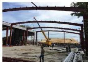
Frame Erection
