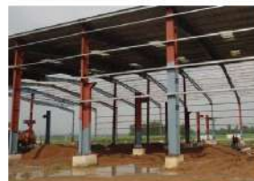
Installation of panel and accessories
